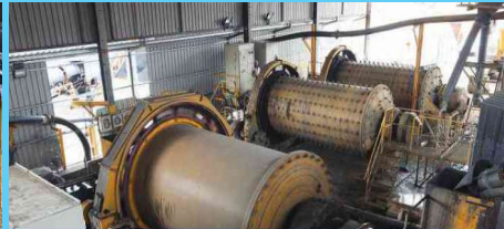
The processing plant
