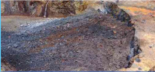
Rock surface after blasting
