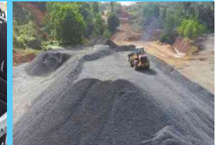
Iron ore fine/lump stockpile
