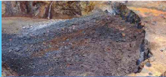
Rock surface after blasting
